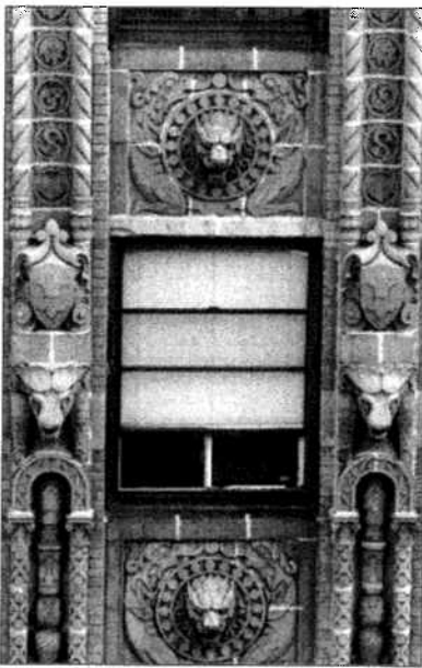
Terra cotta spandrels and exotic ornament supporting the upper parapet.
